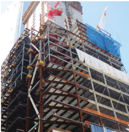
The steel-framed WTC 3, under construction.
