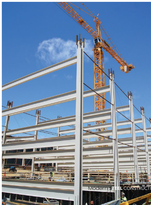
▲ ▼ Braced framing (above) in the new Lot 6, which is eight stories tall and can accommodate 730 cars. It was built adjacent to the existing Lot 5.
