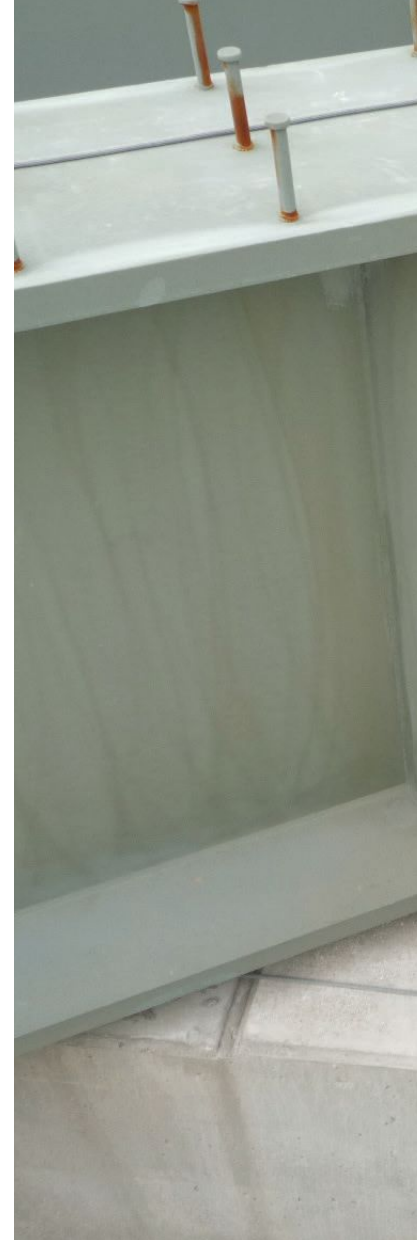
◀ A newly developed split-pipe bearing stiffener (SPBS) connection.
