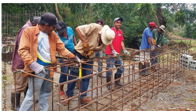
◀ B2P staff and community members assemble the reinforcing cage for the anchor.
